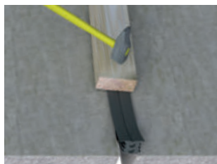
The profile is then pressed into the joint with the help of wood facing.
