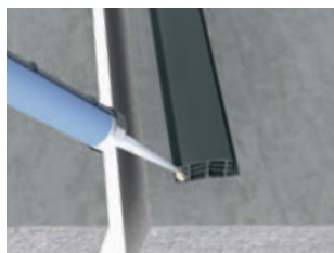
The KP profile is fixed with a neoprene mastic bead applied to the side wings.
